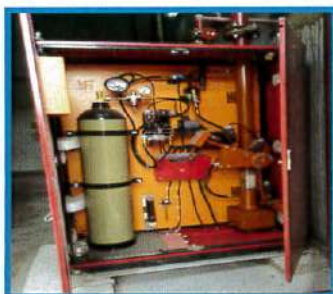
a) Fire Extinguishing Cubicle
