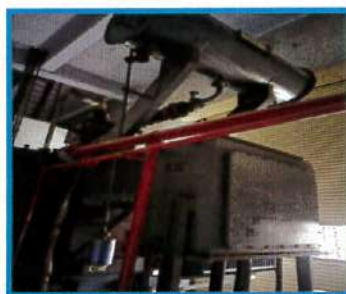
b) Transformer with associated piping and PNRV
