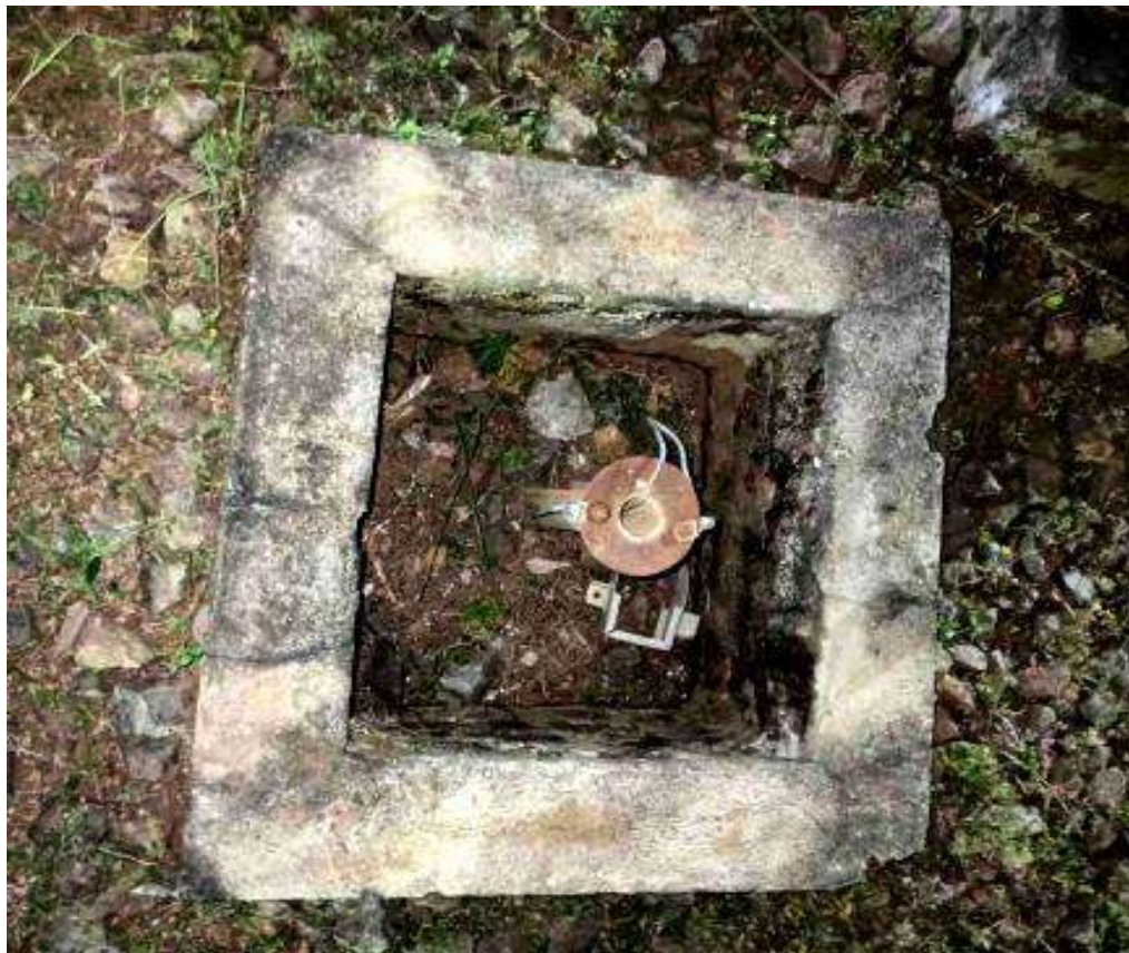
Earthing is done at the PSS, but it is not in good condition.
