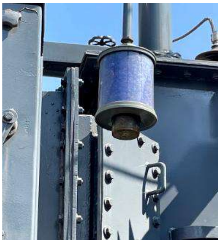
Silica Gel Breather of the Power Transformer is in good condition
