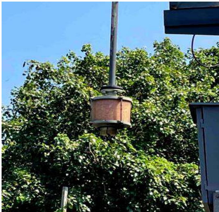
Silica gel Breather of the Transformer is in bad condition.
