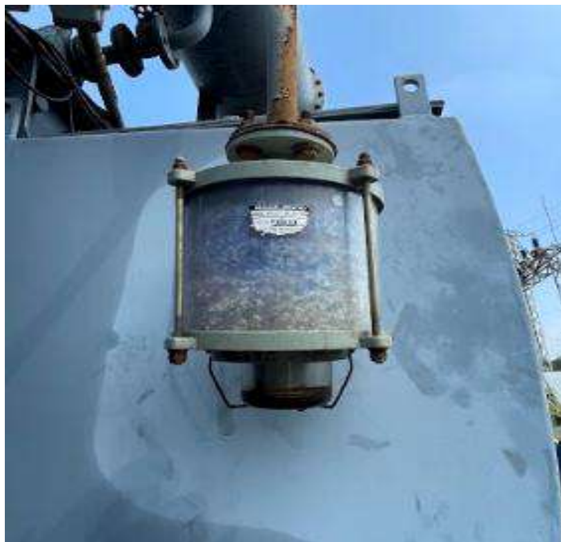
Silica Gel Breather of the Transformer is in good condition
