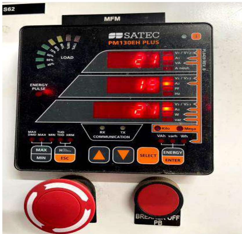
Energy Meter in the Control Panels
