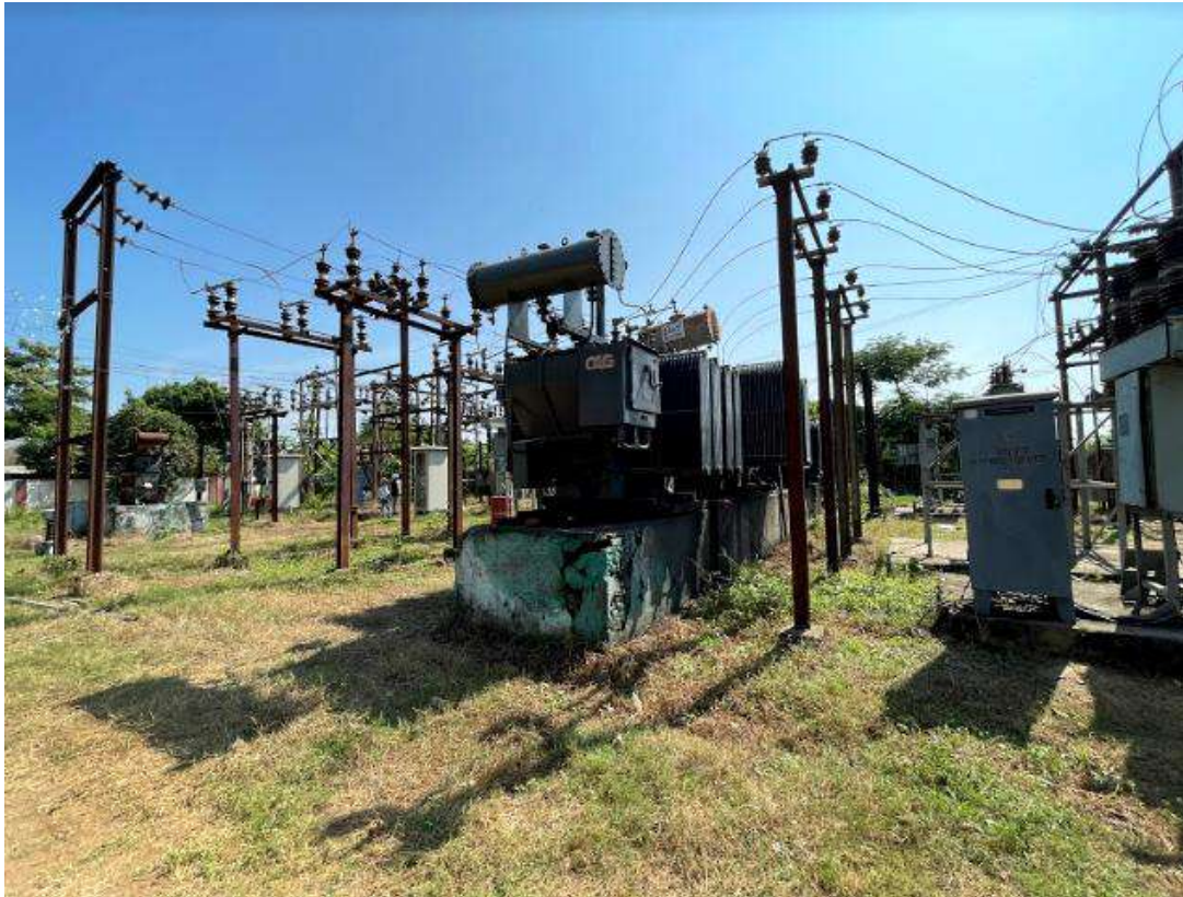
Metal Spreading is not done at the PSS
