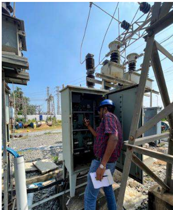
Energy Meter Verification at the PSS
