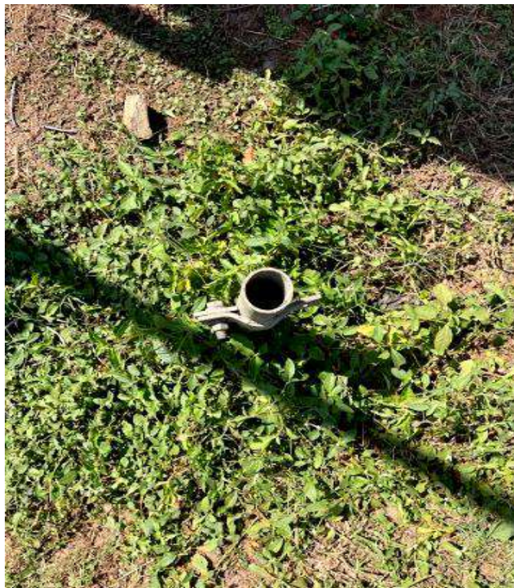
Earthing of the PSS is in bad condition
